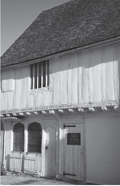
Fig. 1.4. 26 Market Place, Lavenham. Built c.1500 as a domestic house, with a shop occupying the front room of the ground floor. The stall boards visible here may originally have been on the inside, forming a counter, moved outside at an unknown date. The building was later converted into a pub and later still (c.1855) a chapel. It is now a National Trust tea rooms.
